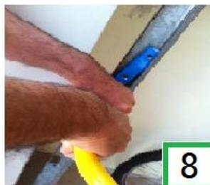
For Added Twisting Power, Use Garage Door Roller Track or Vise
